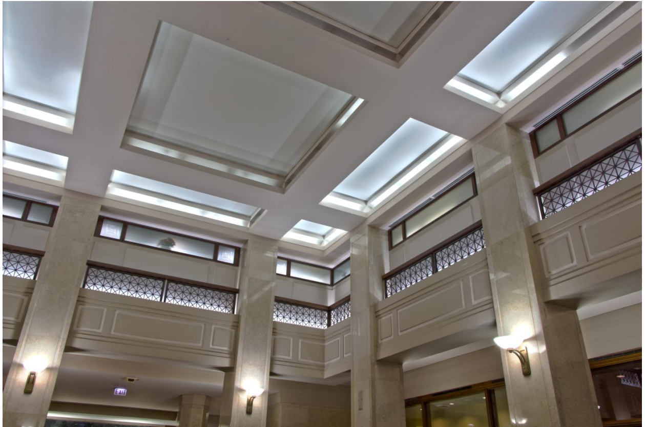
Fig. 13. Burnham Center Ceiling
